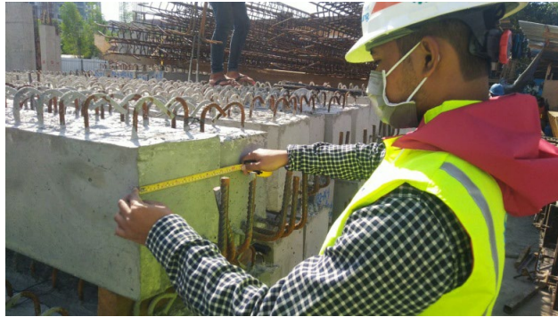
Figure 25: Precast beam dimension checking
