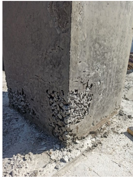
Figure 6: Column casting results
