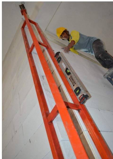
Figure 22: Finishing installation process
