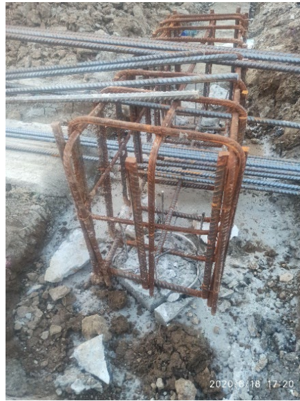
Figure 8: Iron installation before casting
