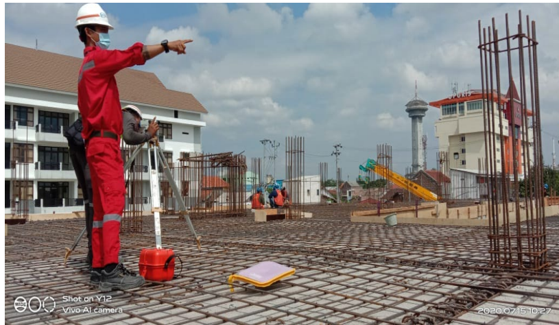
Figure 23: Preparation by safety team
